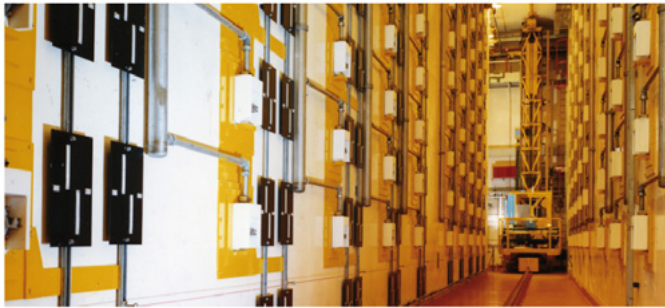
Figure 3: Image of the charge face wall within the charge corridor of a typical SNM store
